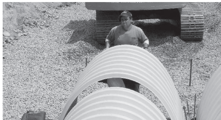
Continue installing chambers by overlapping chamber end corrugations. Chamber joints are labeled "Lower Joint – Overlap Here" and "Build this direction – Upper Joint". Be sure that the chamber placement does not exceed the reach of the construction equipment used to place the stone. Maintain minimum 9" (300 mm) spacing between rows. For the Isolator Row place two continuous layers of ADS Woven fabric between the foundation stone and the isolator row chambers, making sure the fabric lays flat and extends the entire width of the chamber feet.
